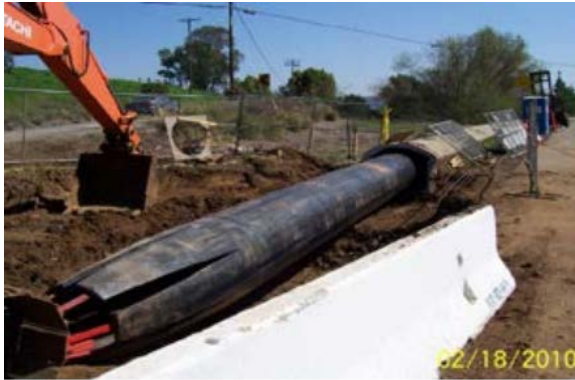
Rehab HDPE Line
