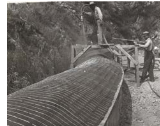
VID covered seven miles of open flume from 1947 to 1955
