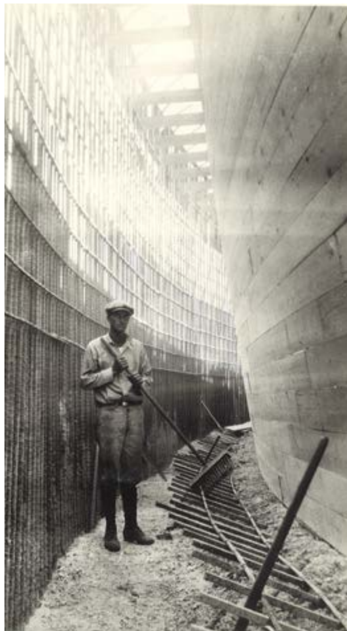
Construction of Henshaw Dam, 1922
