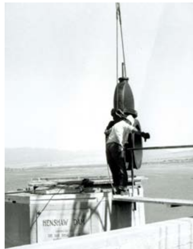
Replacing outlet valve at Henshaw Dam, 1959
