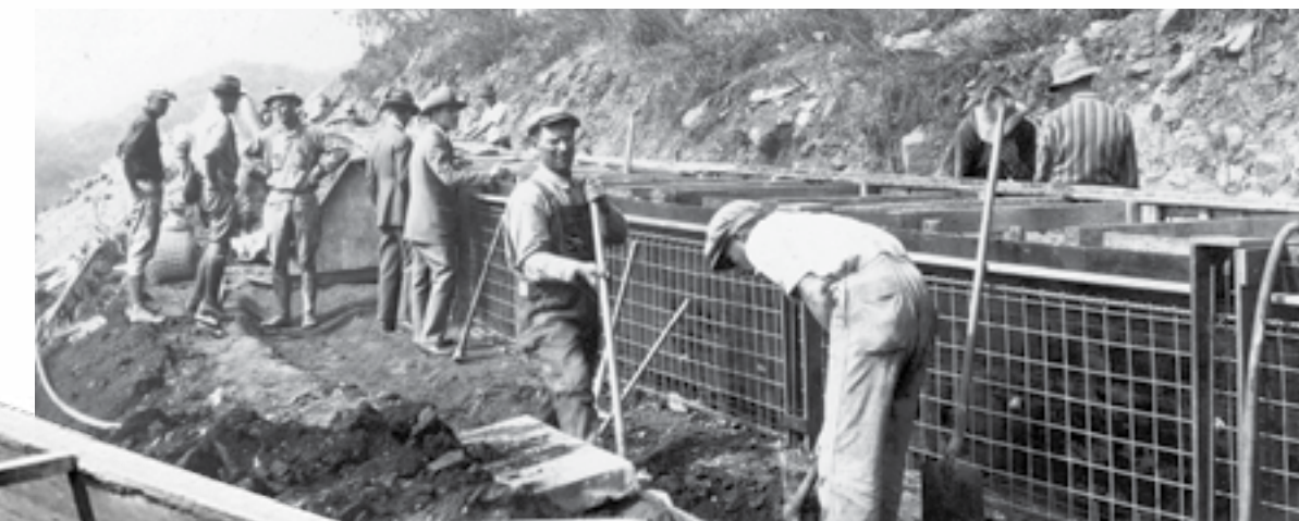
Big Tunnel Bench construction, 1925
