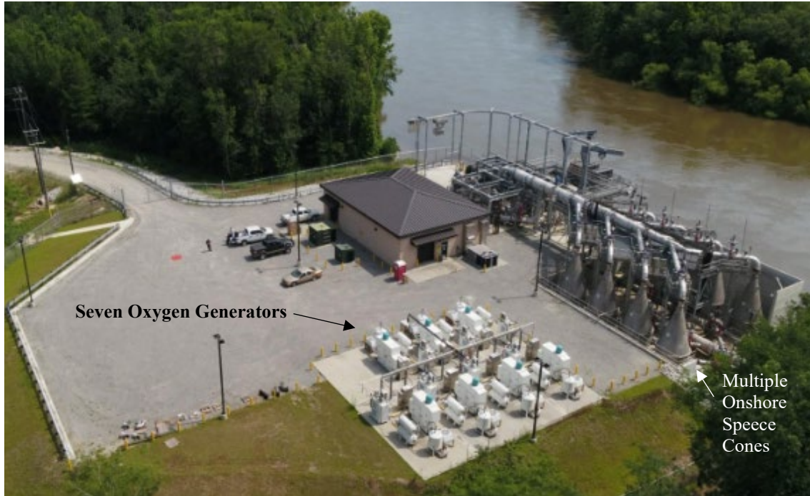
Figure 4-14. Example oxygenation system with onshore Speece cones and oxygen generators. Photo Reprinted from US Army Corps of Engineers Startup Run Data Collection & Modeling Report , Oxygen Injection System Environmental Testing for the Savannah Harbor Expansion Project, March 2021.
