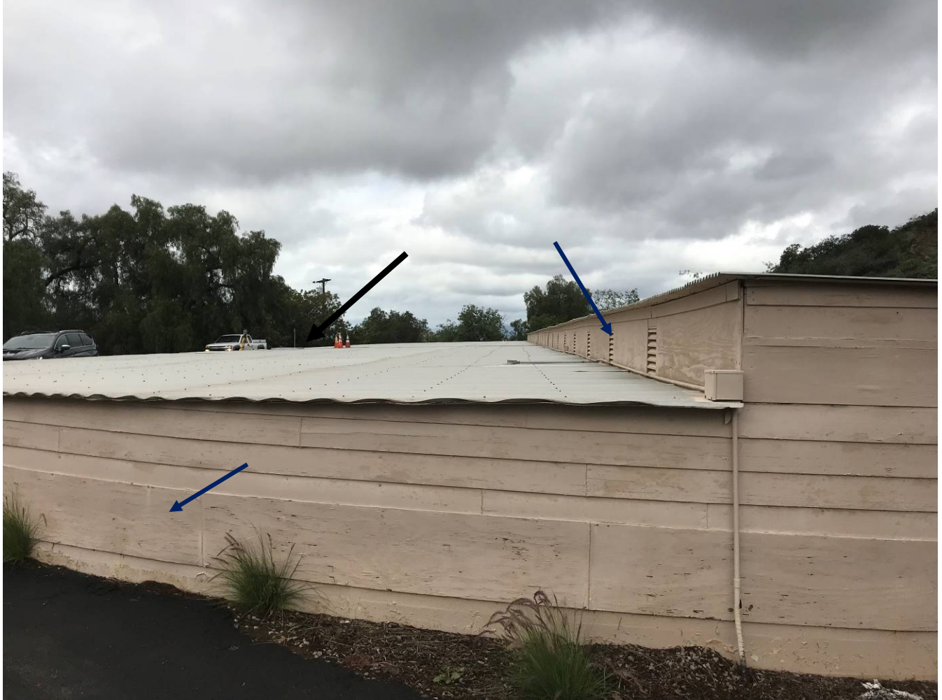
Photo Three: Ground level photo of Edgehill Road Reservoir. The blue arrows point to the plywood over the screens around the perimeter of the tank and the louvers on the center area of roof. The black arrow points toward the access hatch used to enter the tank.
