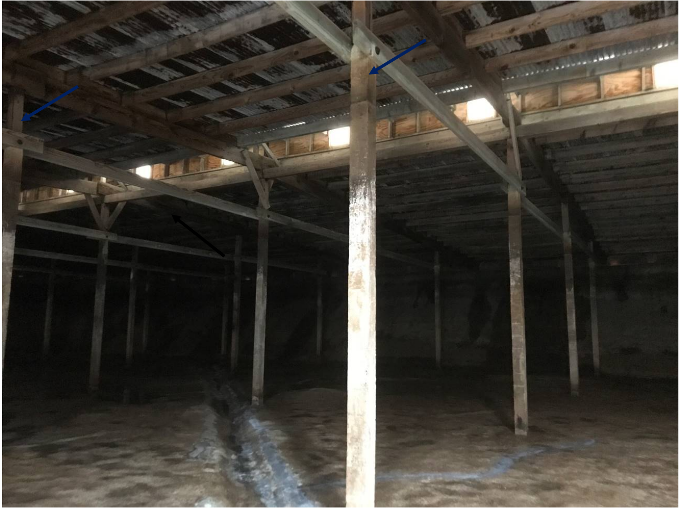
Photo Five: The blue arrows point to the wood framing on the interior of the tank above the concrete columns.
