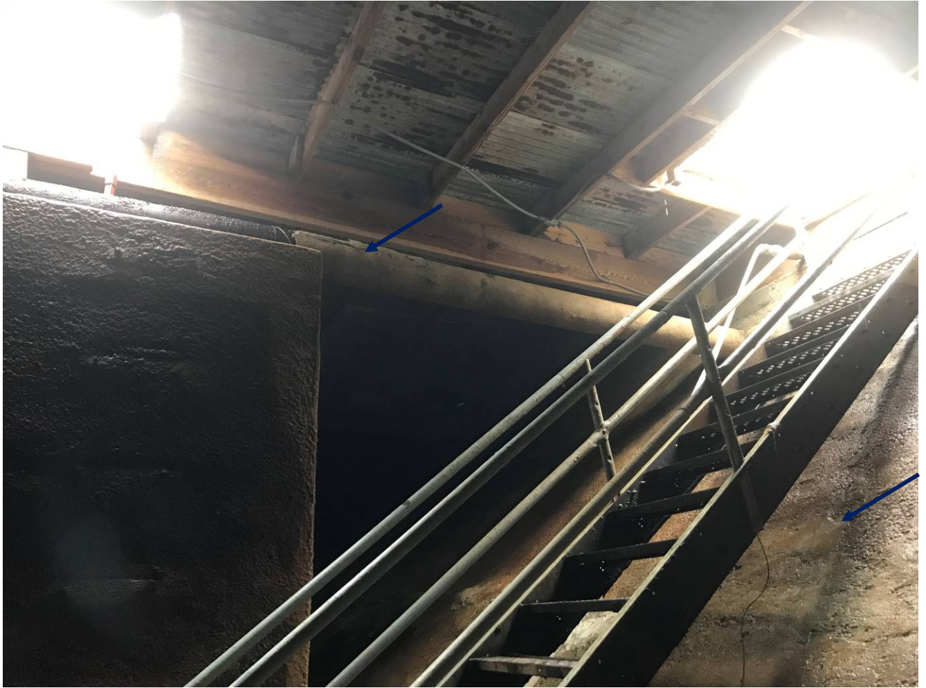
Photo Four: The stairs inside the tank looking towards the access hatch. The arrows point to the inlet pipe and the gunnite on the interior walls,
