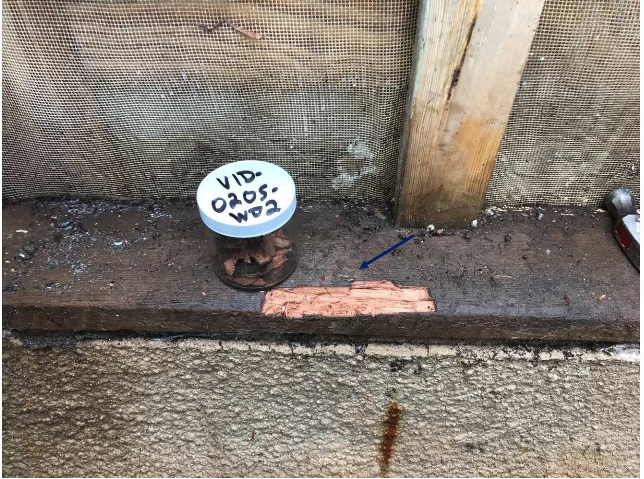
Photo Six: The bottom plate on wall around the perimeter of the tank.
