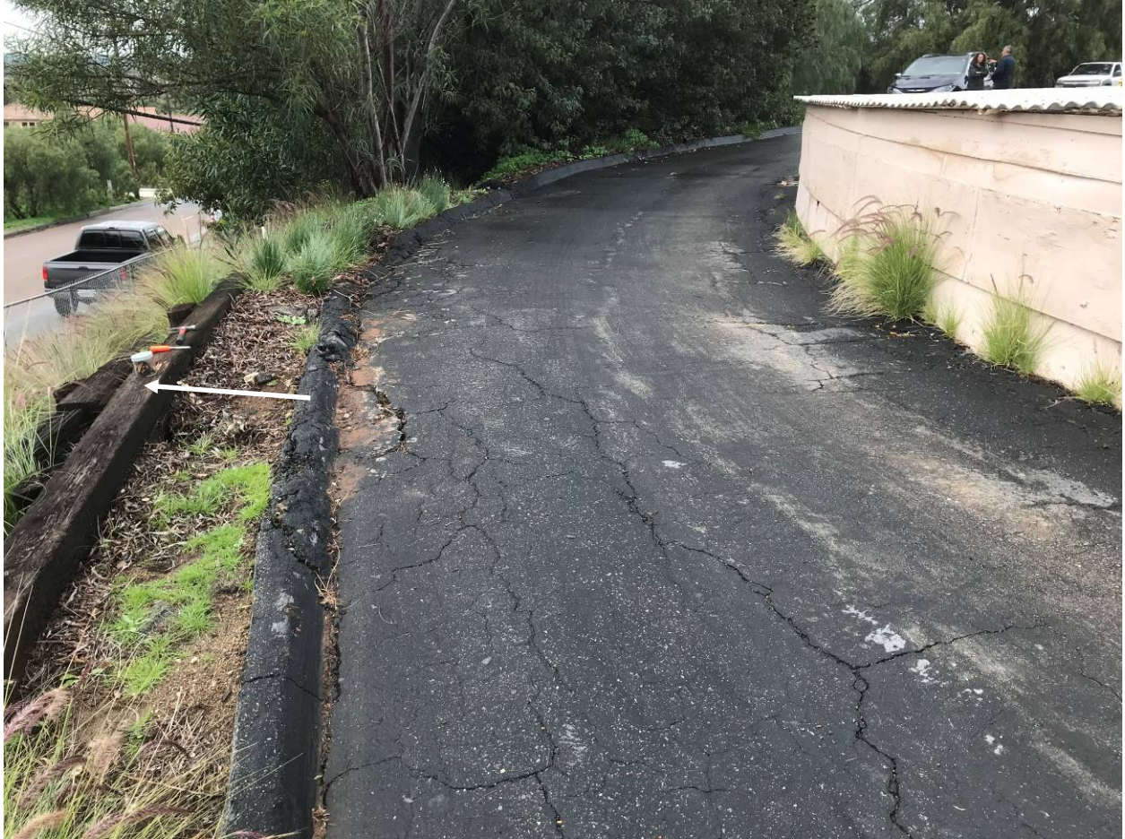
Photo Seven: The arrow points to the railroad ties that were tested on the outside of the tank.
