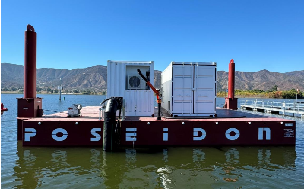
Figure 4: System Installation Picture
