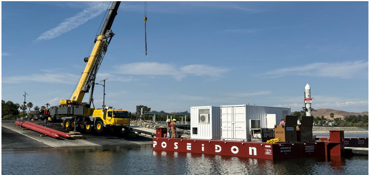
Figure 5: Crane Placement of Container on Barge
