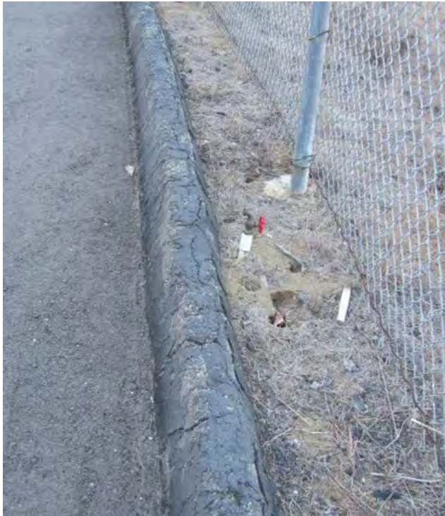
Figure 4-3. Pavement Cracks
