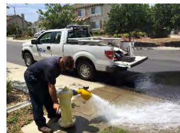
Residual Hydrant 13124 (Test 17)
