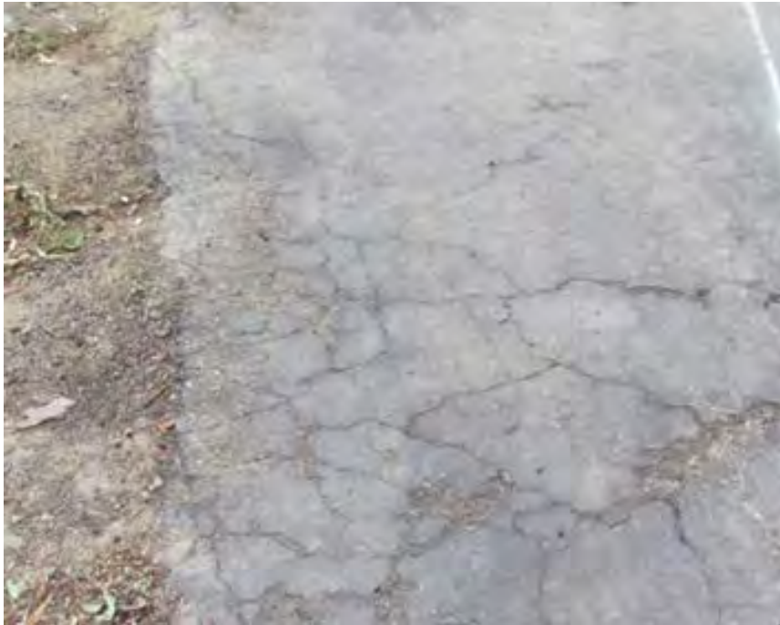
Figure 5-4. Pavement Cracking
