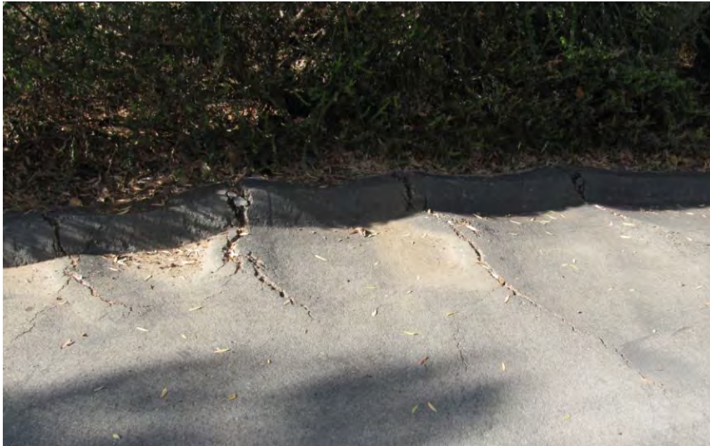
Figure 9-4. Pavement Cracks
