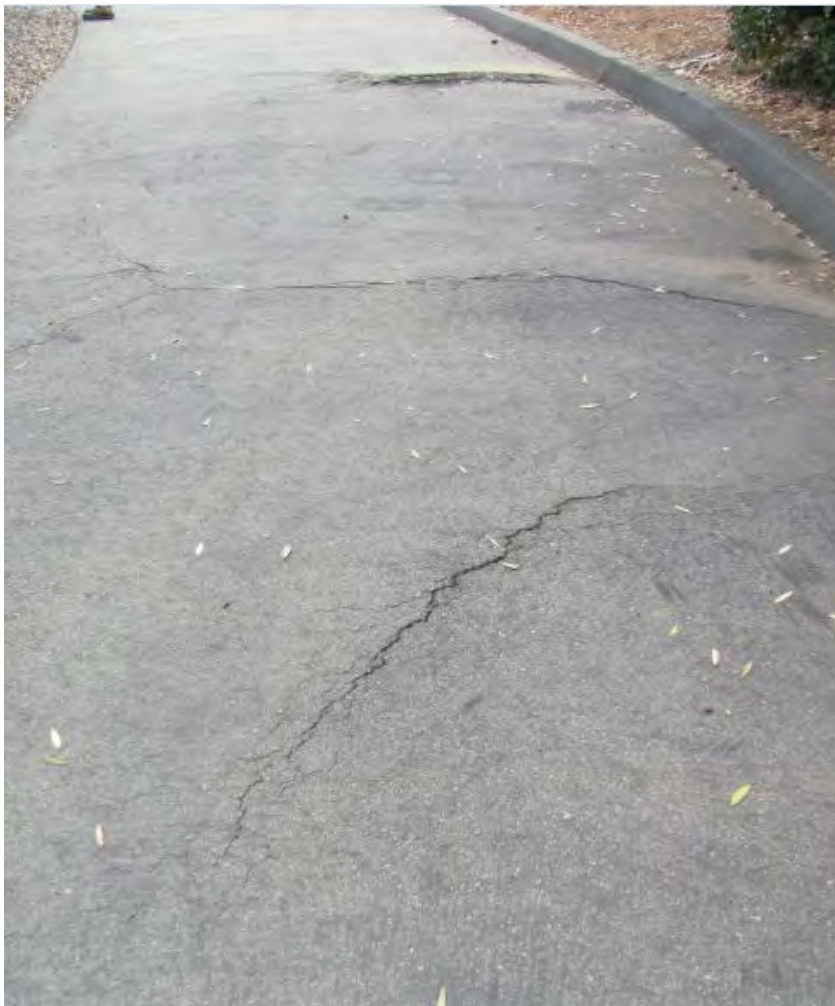
Figure 9-4. Pavement Cracks
