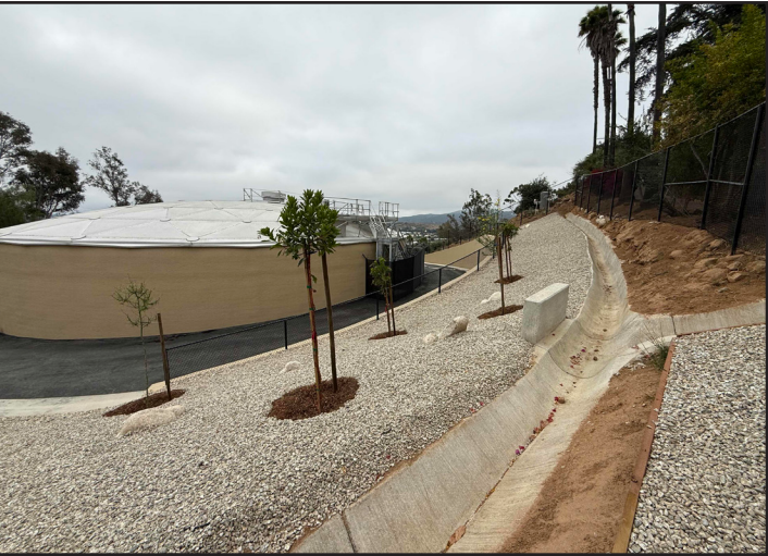
ABOVE: Completed rehabilitation project
