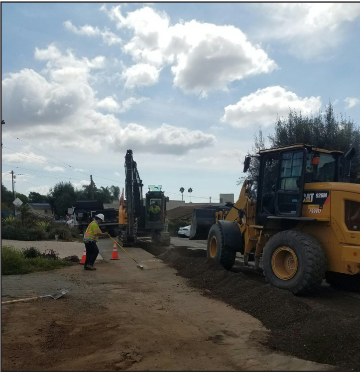
ABOVE: Independence Way mainline replacement construction
