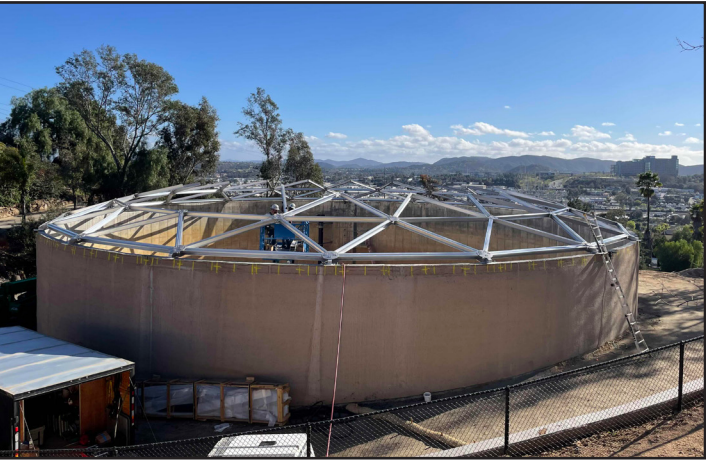
ABOVE: Construction of new roof
