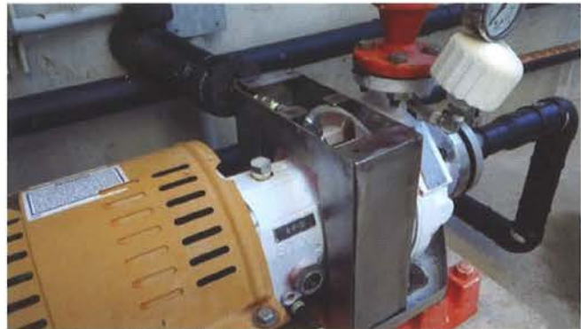
Central Coast Water Authority – Maintenance staff at the water treatment plant fabricated a splash shield to prevent contact with caustic soda solution during a seal flush of the suction pump.
