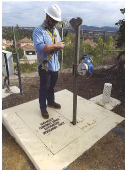
Vista Irrigation District – The district cut a small opening in the vault lid directly above the fall protection receiver and installed a hinged cover to secure the opening and the receiver when not in use. The design allows the davit arm to be attached to the receiver and the employee to be tied off prior to the vault lid being opened.
