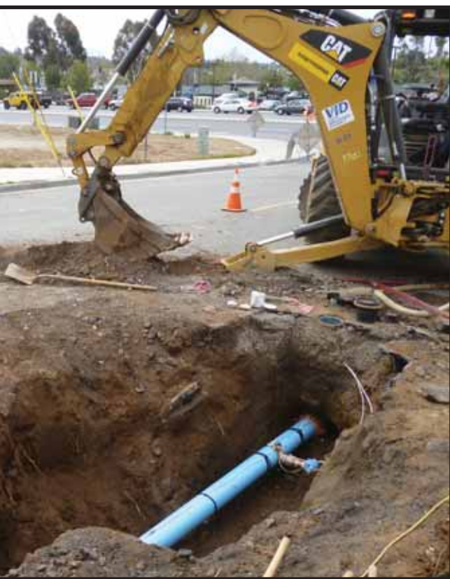
Installation of an 8" C-900 PVC pipeline in North Santa Fe and Washington Street in Vista.
