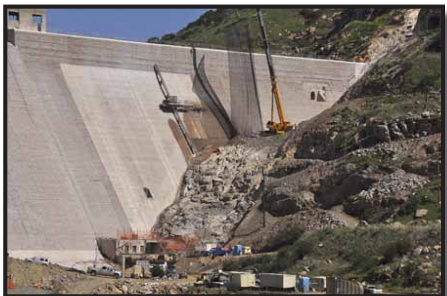
San Vicente Dam under construction
