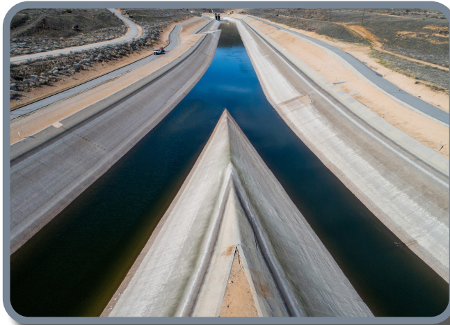
Purchased Water Source: California Aqueduct Photo Credit: Ken James, DWR
