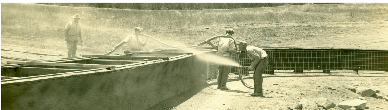
Gunnite process along Vista Flume 1920's
