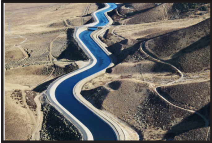
Imported Water Source: California Aqueduct
